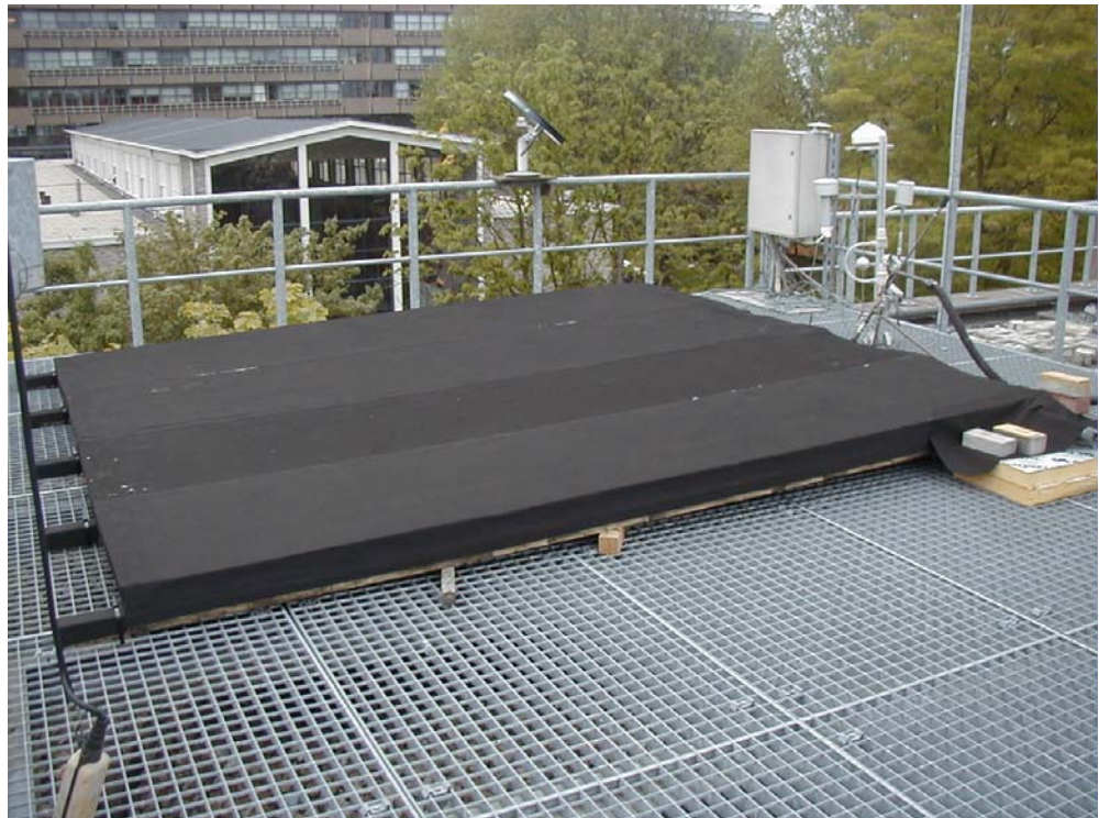
Figure 1: Collector during test on roof
